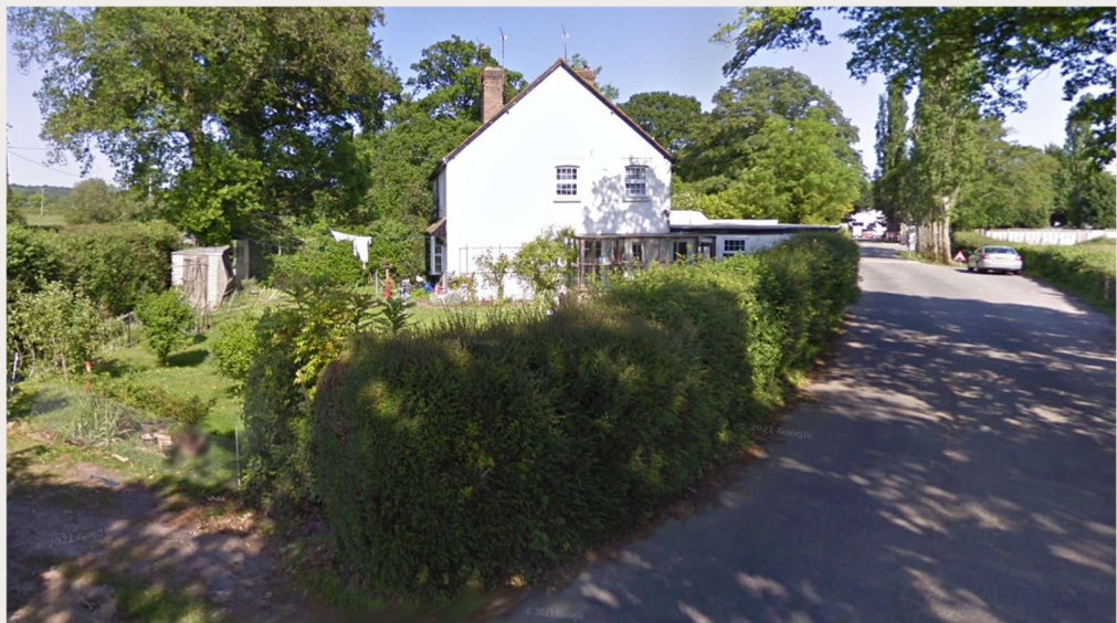
Image capture: July 2009 © 2024 Google. Above 'Adjacent property'
